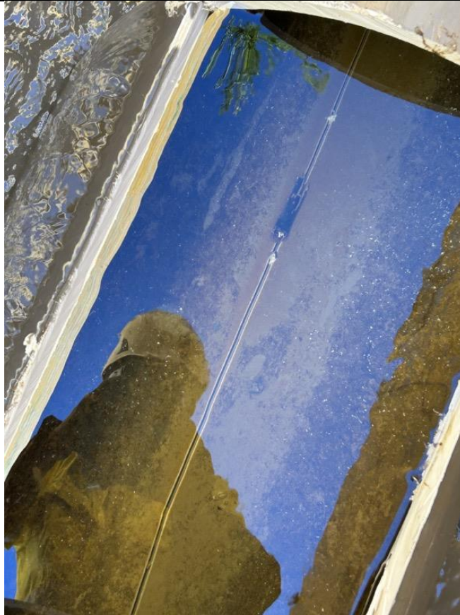
Longitudinal split in existing line (pipe crown removed)
