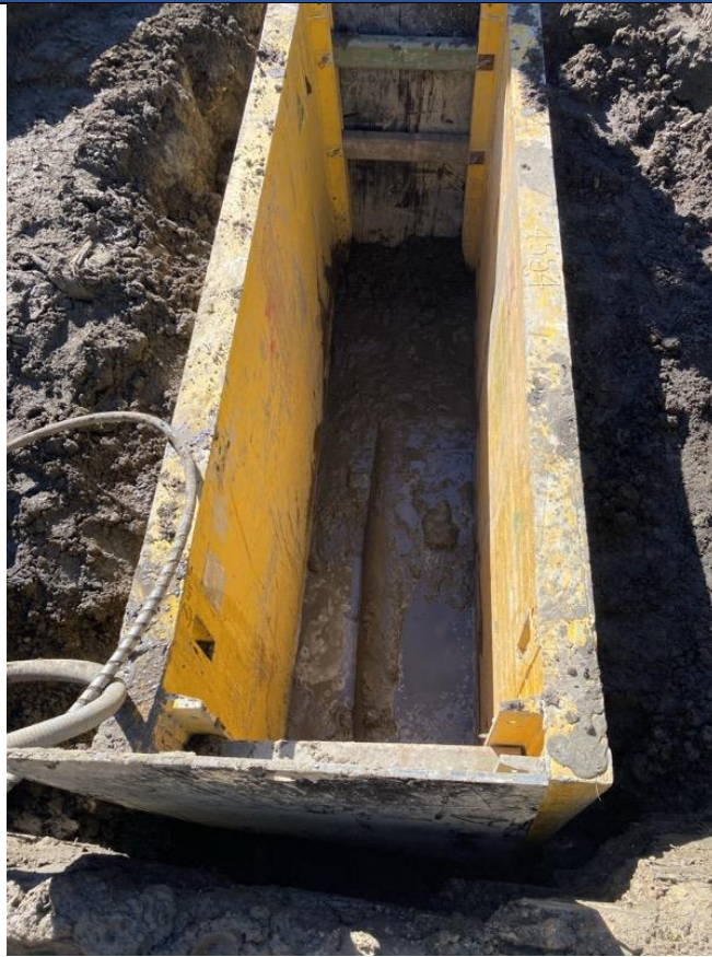
Excavation exposing top of recycled water line
