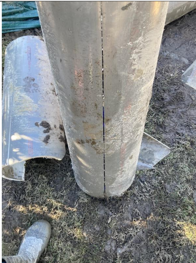
Longitudinal split in existing line
