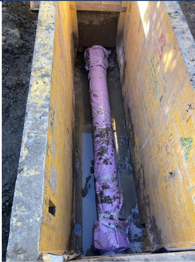
Completed repair wrapped recycled water line
