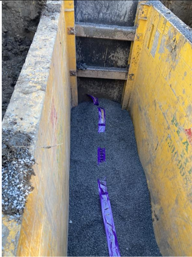
Repaired line in screening s with detectable tape
