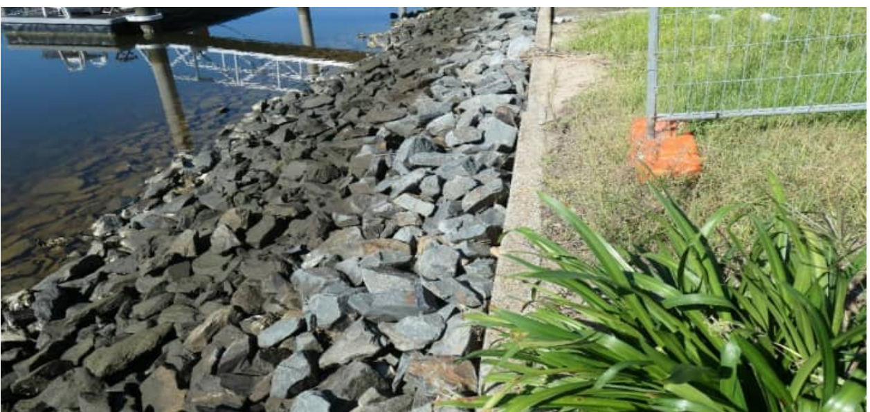
SCE-06: example view of gabion rock armour profile
