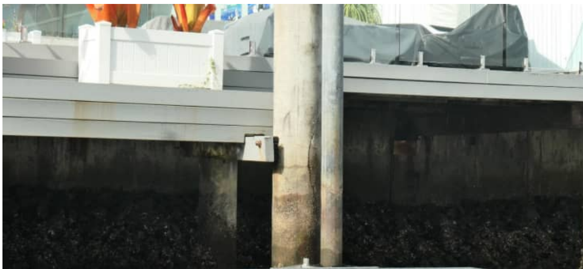
SR-24: spalling damage repairs required to 5662 Harbour Tce mooring pile
