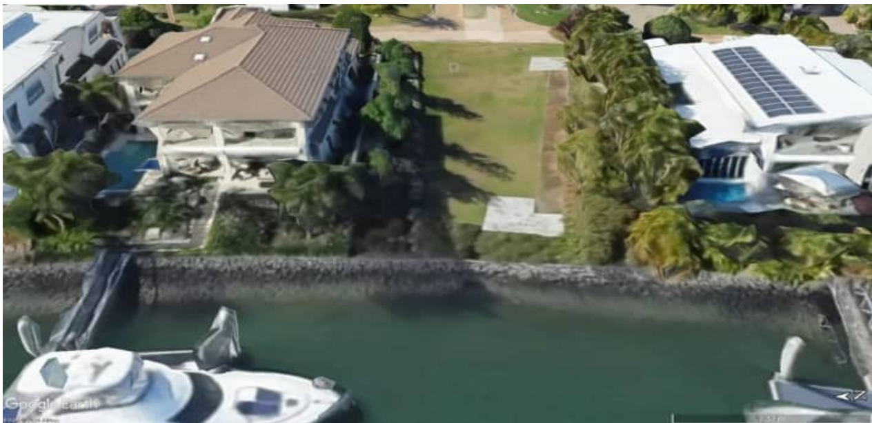
SCC-05: RCP drainage / headwall outlet off The Circle
