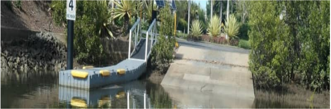
SR-50: boat ramp and polyethylene finger pontoon adjacent to The Parkway
