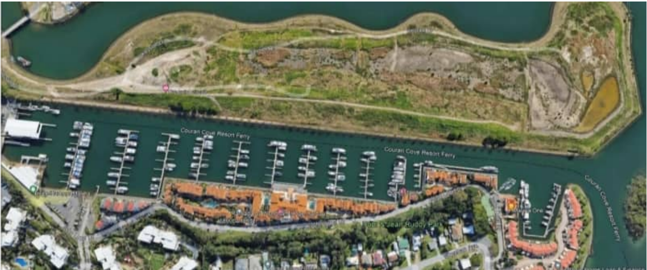
SR-74: overview of The Point Cct
