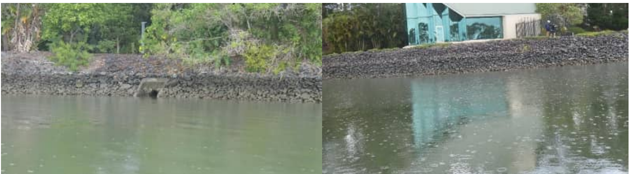
SR-16: example views of Harbour 1 revetment wall / edge treatment (good) condition – #2
