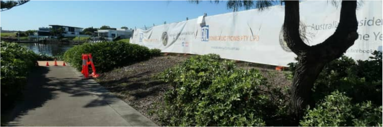
SCE-04: typical view of easement arrangement
