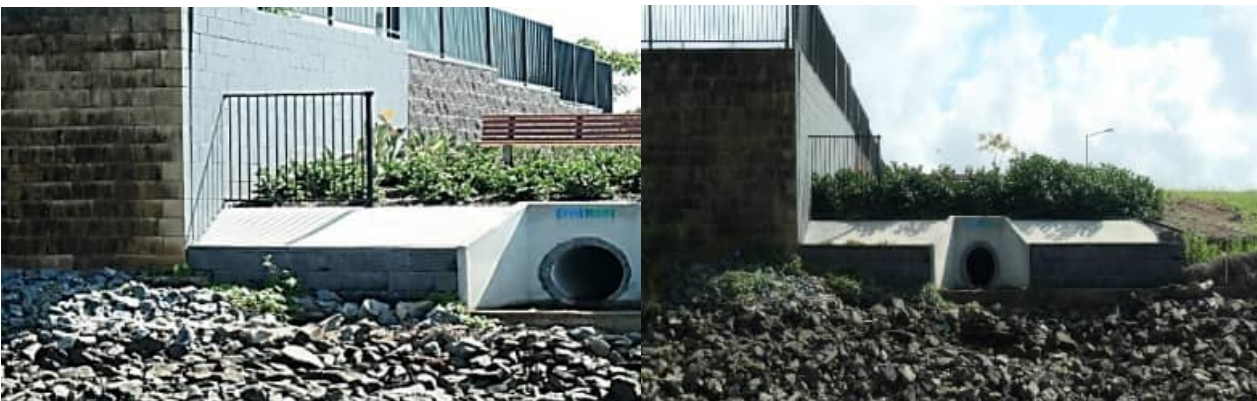
SR-75: comparison views of rock armouring condition at the SW outflow off The Point Cct (LHS = 2023 / RHS = 2024)
