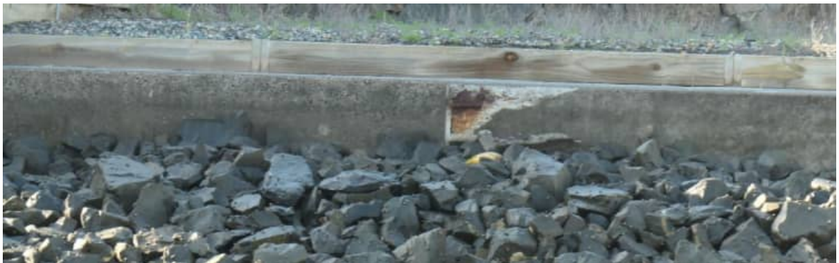
SR-06: spalling damage to revetment wall arrangement (circa) 5240 Marine Dve Nth
