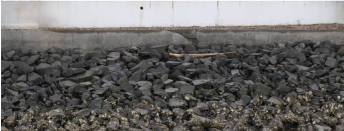
SR-30: revetment wall arrangement stem spalling damage at 5715 Anchorage Tce
