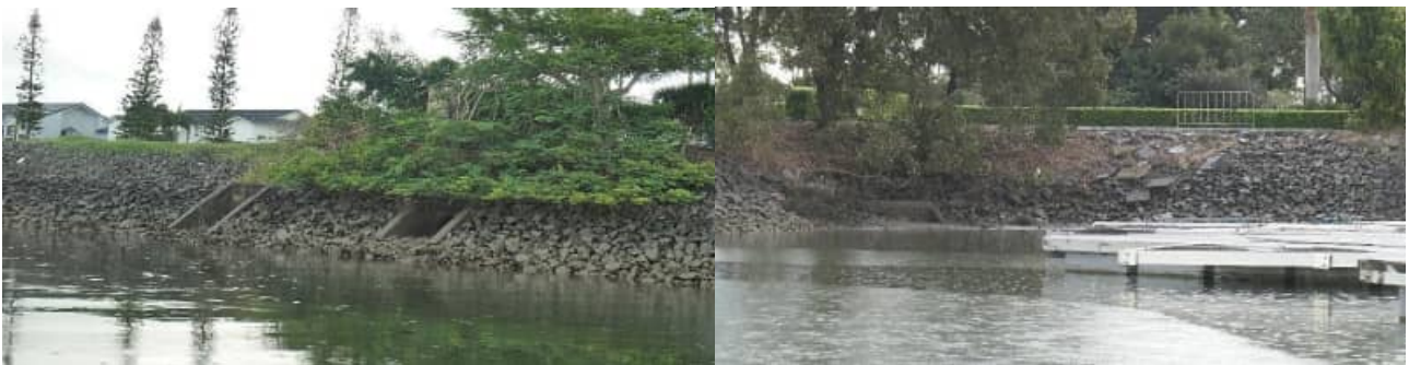
SR-15: example views of Harbour 1 revetment wall / edge treatment (good) condition – #1
