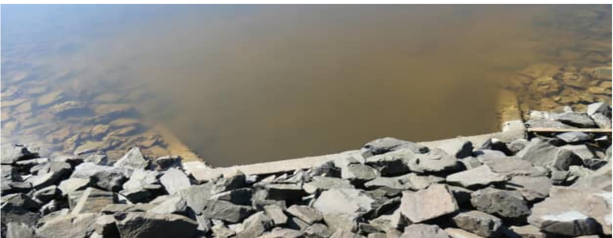
SCE-05: example view of reinforced concrete headwall
