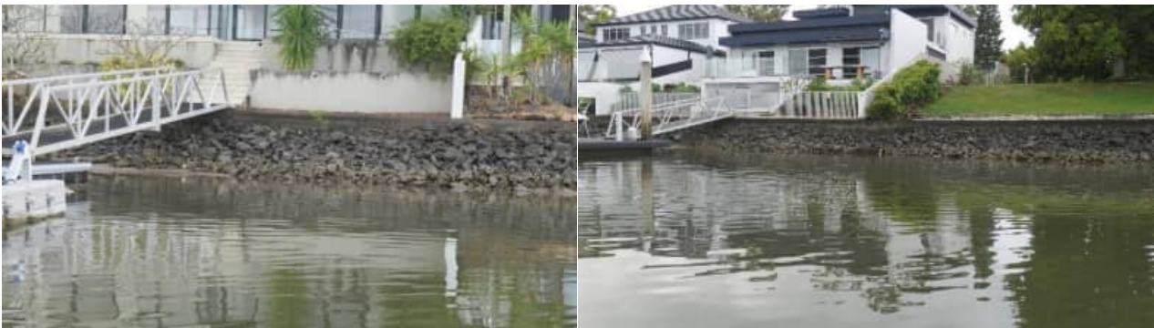
SR-04: Typical revetment wall arrangement (good) condition along Marine Drive North
