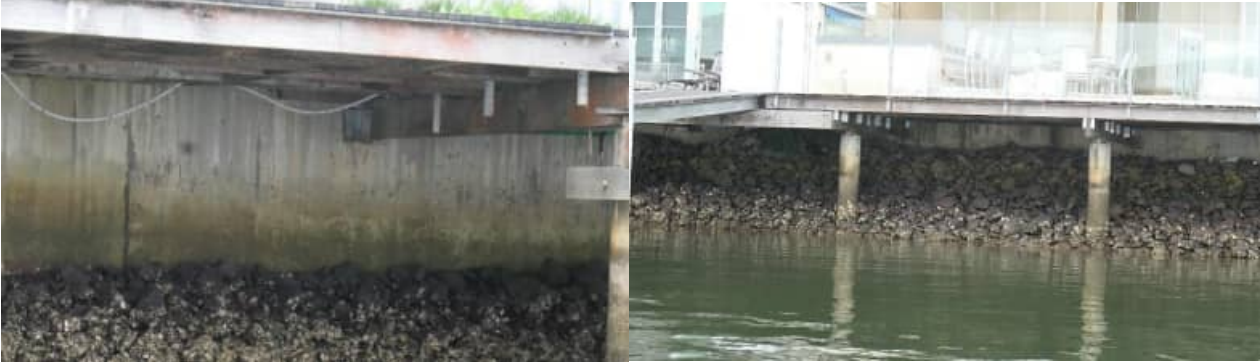
SR-19: example views of Harbour 1 revetment wall / edge treatment (good) condition – #5
