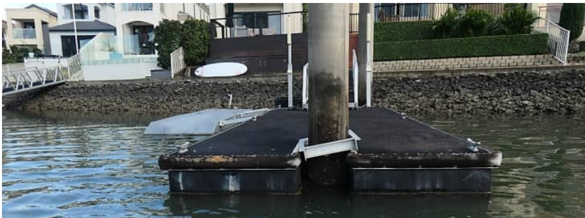
SR-56: view of compromised finger pontoon mooring bracket at (circa) 8047 The Parkway
