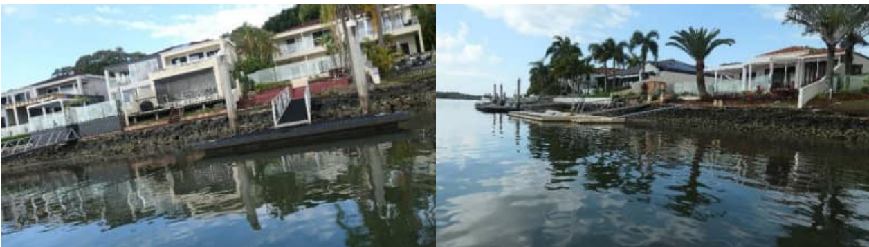
SR-44: example views of generally good condition of revetment wall arrangement / rock armouring to 'Plumeria' - #2
