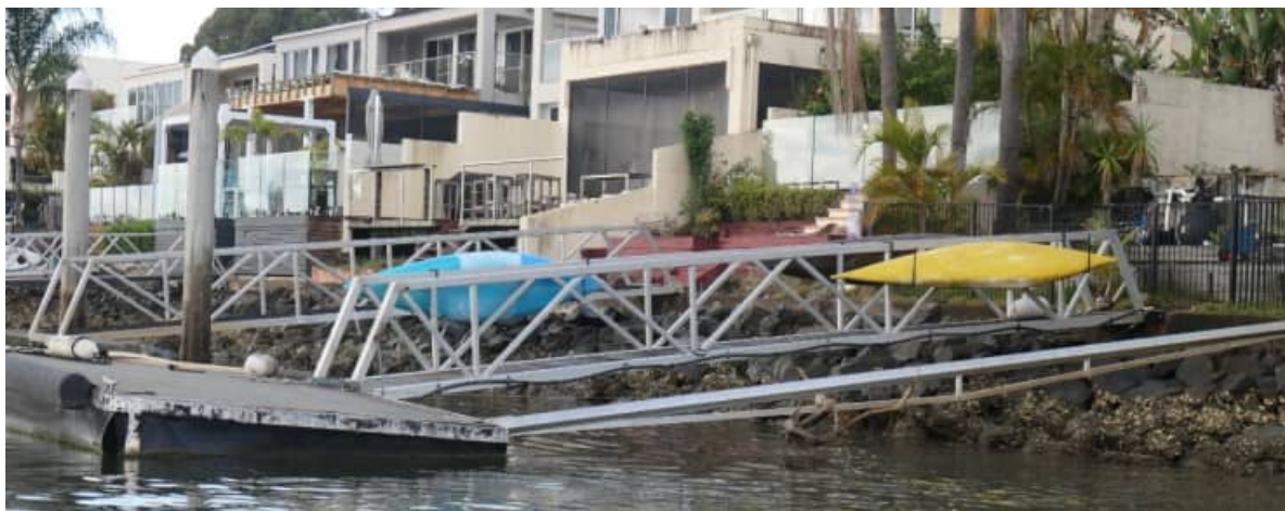
SR-46: view of compromised pontoon at 7100 Marine Dve East - #1
