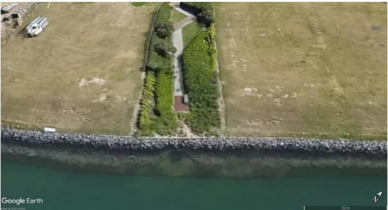
SCE-03: RCP drainage / headwall outlet
