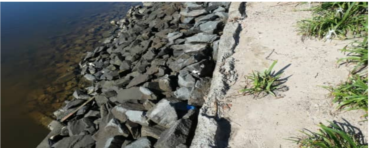
SCE-08: example view of stem deterioration to revetment wall arrangement at easement - #1
