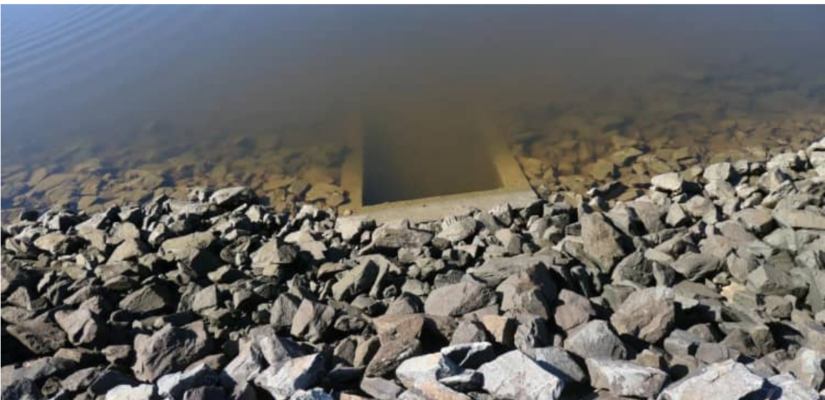
SCE-07: example view of reinforced concrete headwall
