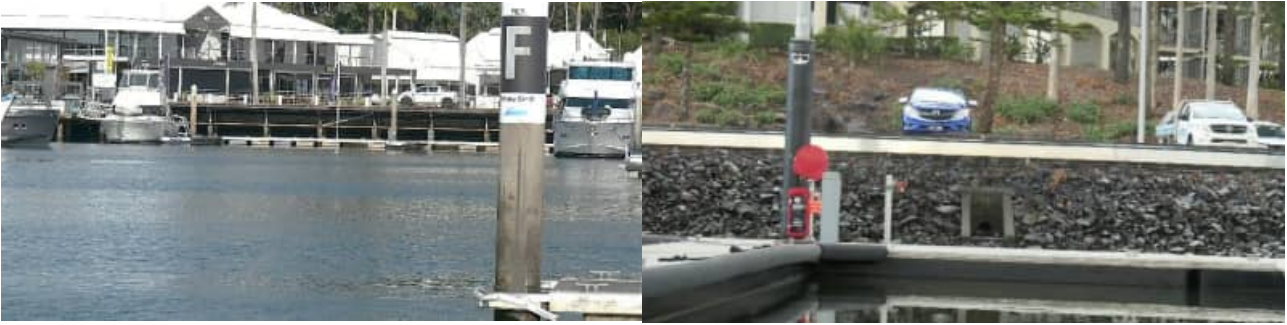
SR-17: example views of Harbour 1 revetment wall / edge treatment (good) condition – #3
