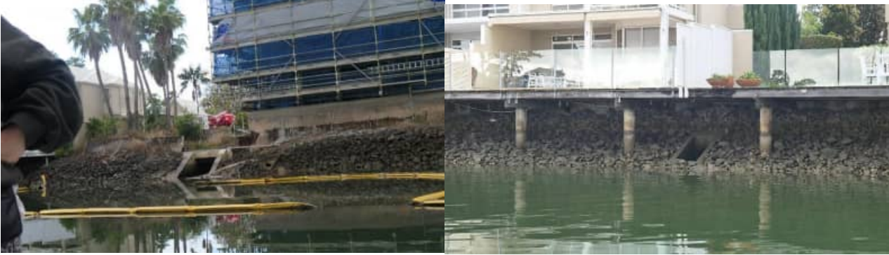
SR-18: example views of Harbour 1 revetment wall / edge treatment (good) condition – #4
