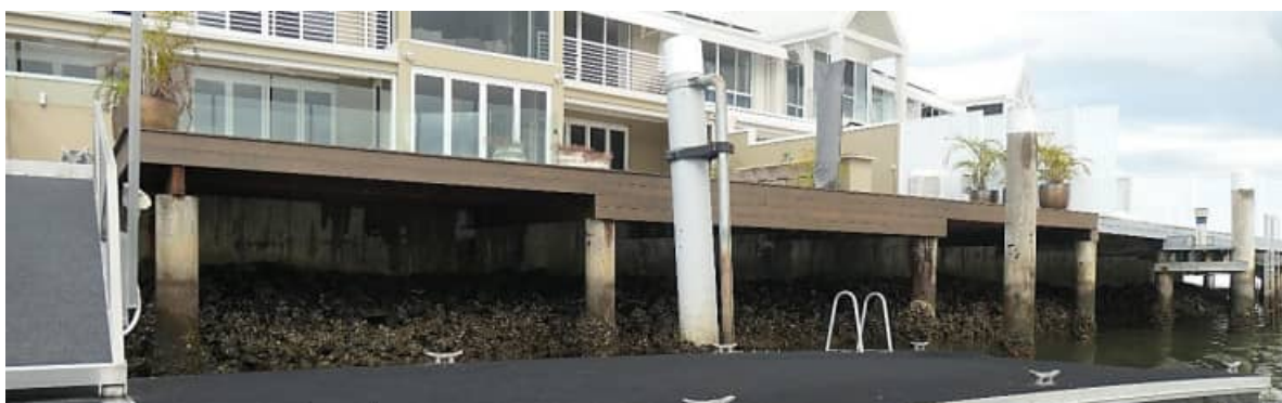
SR-25: realignment of unacceptably off-vertical restraint pile to required to 5670 Harbour mooring arrangement
