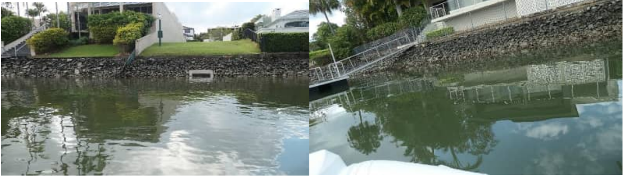
SR-36: example of HBR-2 revetment wall and rock armouring (good) condition – #3
