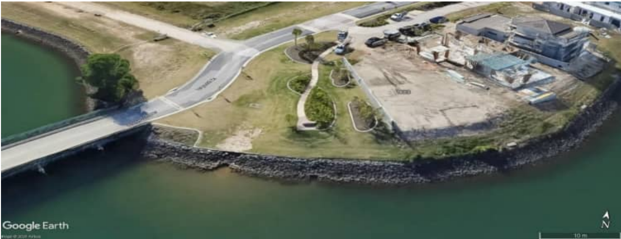
SCB-01: overview of easement between the 'Sickle Ave' bridge and Lot 1080 Edgecliff Dve
