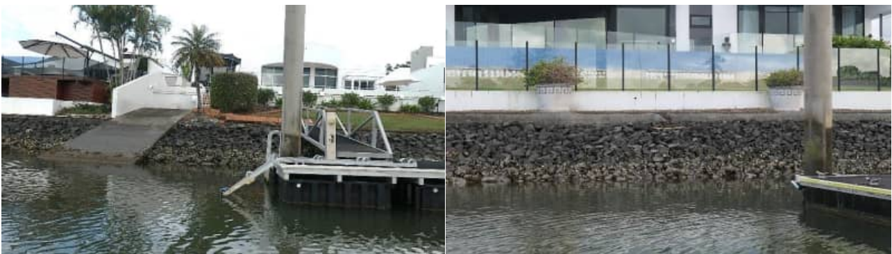
SR-29: example views of Coomera River ('Bauhinia') revetment wall and rock armouring (good) condition – #3
