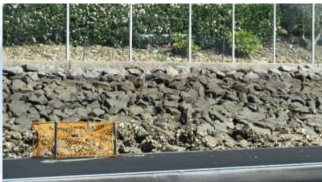
SR-61: example views of typical revetment wall / rock condition to the 'Schotia' precinct - #1
