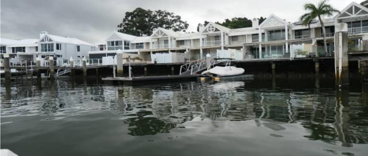
SR-20: example view of Harbour 1 revetment wall / edge treatment (good) condition – #6
