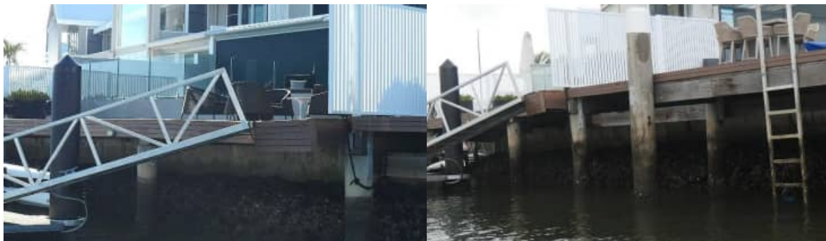
SR-23: potential boardwalk framing failure at 5654 The Parkway
