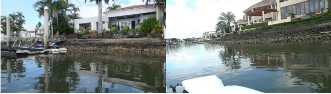
SR-45: example views of generally good condition of revetment wall arrangement / rock armoring to 'Plumeria' - #3
