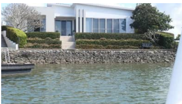
SR-61: example views of typical revetment wall / rock condition to the 'Schotia' precinct - #1
