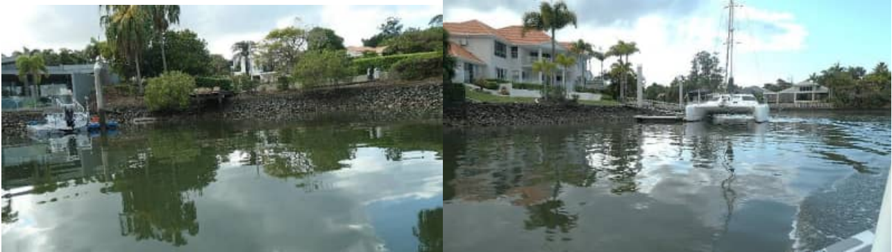
SR-37: example of HBR-2 revetment wall and rock armouring (good) condition – #4
