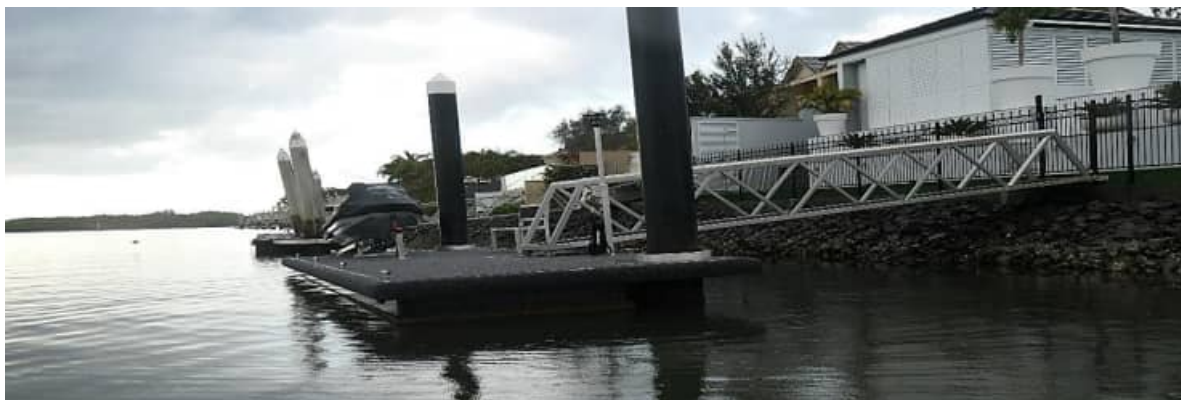
SR-10: off-vertical alignment to pontoon piles (circa) 5320 Marine Dve Nth
