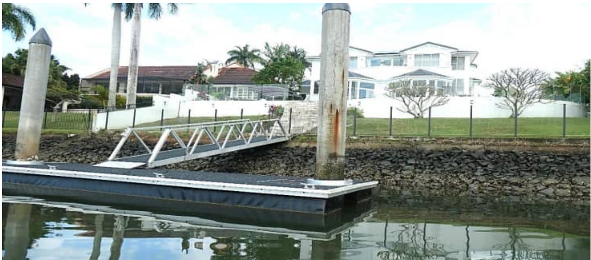
SR-39: mooring pile spalling damage at 5843 Coveside Ln
