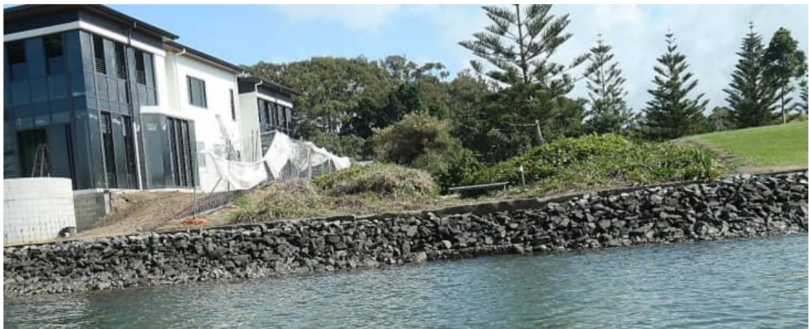
SR-71: damaged revetment wall arrangement to easement between 1044 and 1051 Edgecliff Dve
