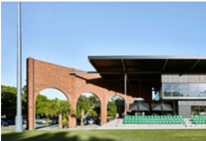
Wests Rugby Club Hutchinson Builders
